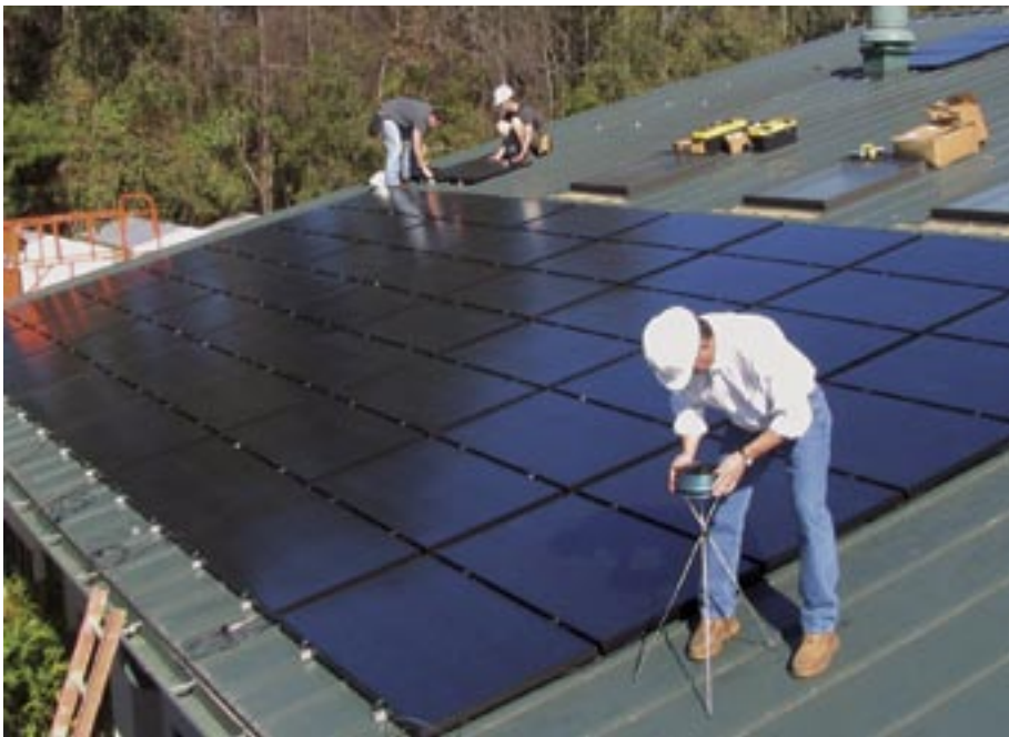
Installation of a 25kW commercial grid-tied PV system in Savannah, GA.
